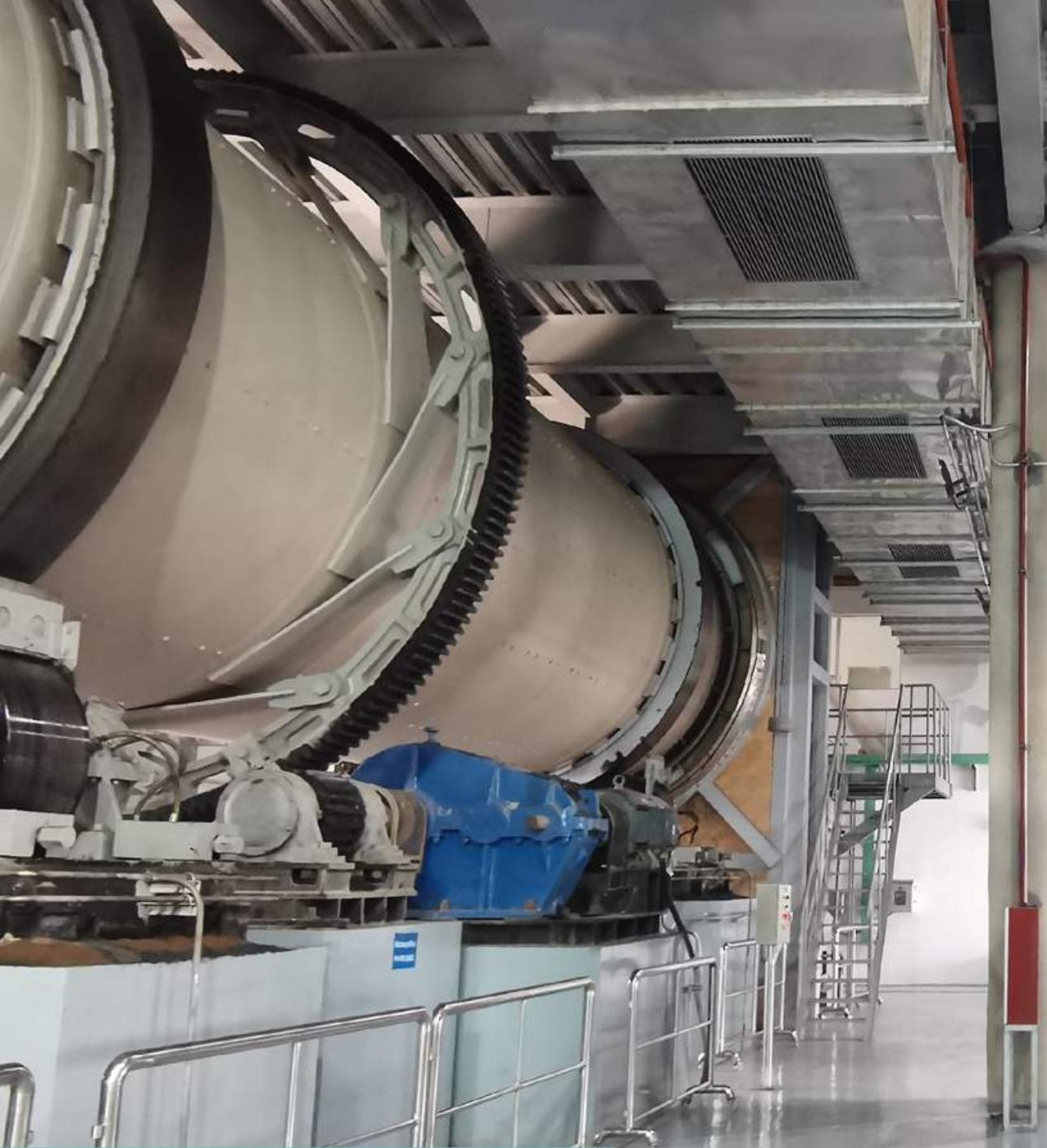
**Primary Combustion Chamber of the Sludge Drying & Incineration Plant of Dasherkandi Sewage Treatment Plant**
