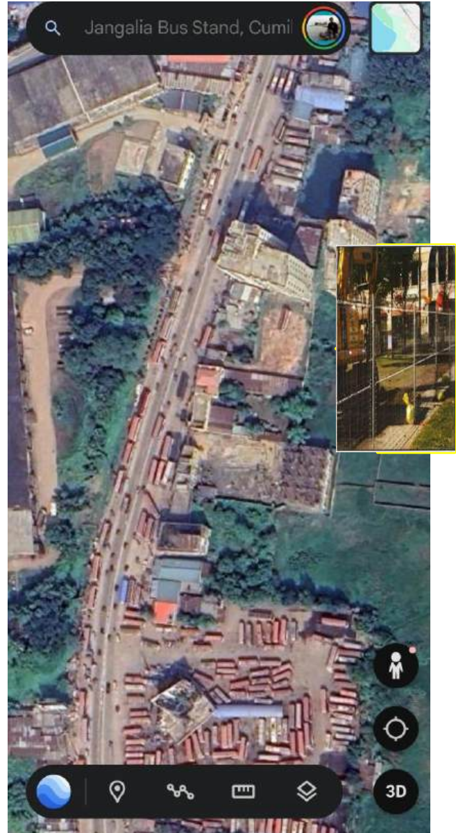
Google Earth view of proposed new OHT construction site at Jangalia CuCC
