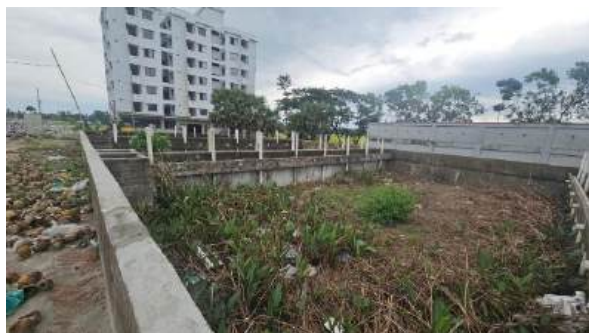
Sewage treatment plant at the North side of the proposed OHT plant
