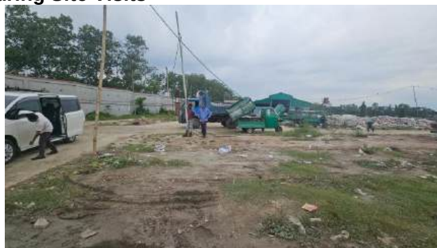
Photo of Southward View of proposed OHT site. Beyond boundary wall is the local Paurashava road connected with town.
