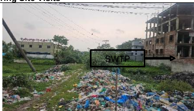
View of the SWTP Hajiganj from the Chandpur Hajiganj Highway which bounds the SWTP by the South side
