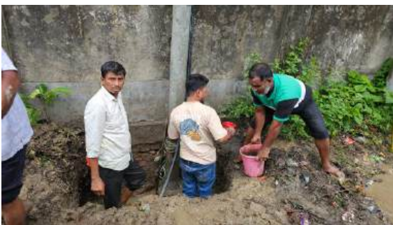
Photo 1: Repairing pipe leakage in Chandpur Paurashava.
