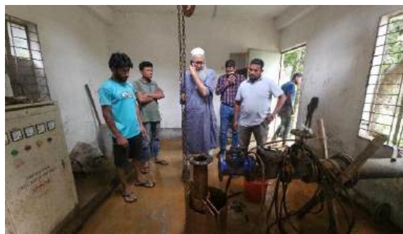
Photo 6: PTW repairing works at Hajiganj.
