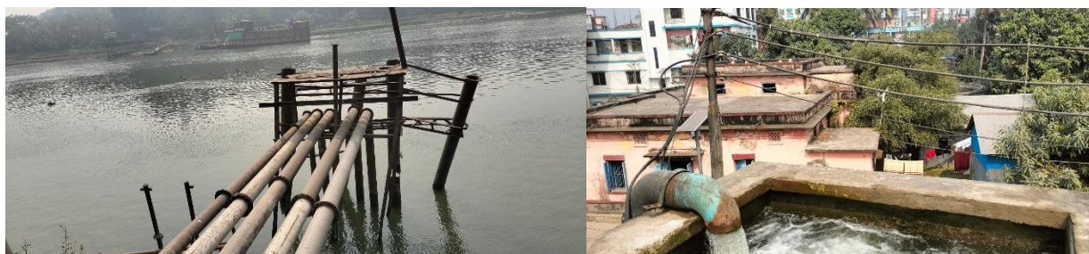
Figure 3: Site inspection and discussion at SWTP
