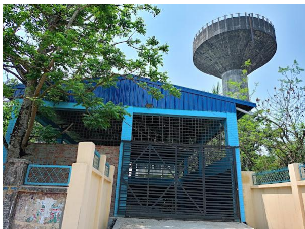
Photo 1: Newly constructed Secondary Transfer Station and the old Water Tank near PTI, Natore.
