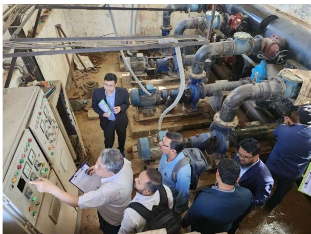
Pic: Site visit for practical training at Sylhet City Corporation WTP
