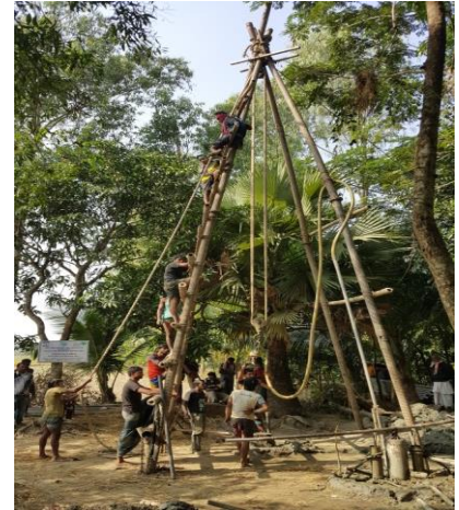
Figure 7: Drilling of Test Well
