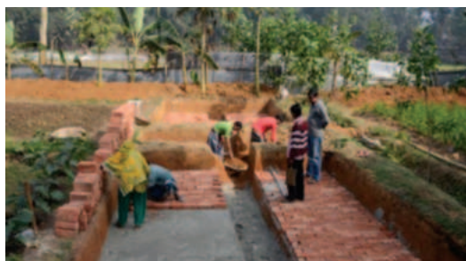
(a) Drying beds - masonry work
