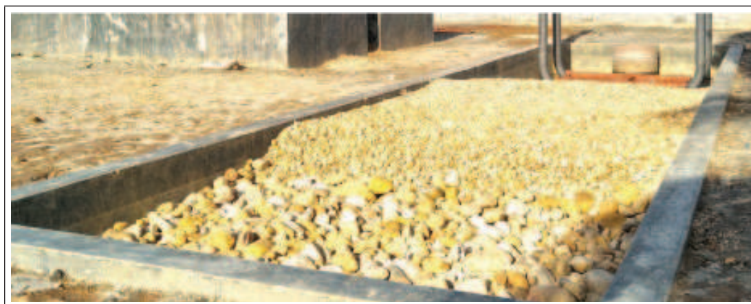
Figure 27: Construction of Planted drying bed at Mymensingh City Corporation, FSTP.
