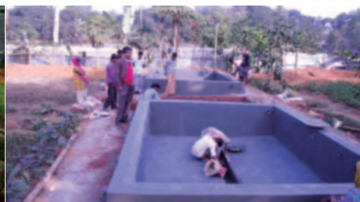
(b) Drying beds - plastering work
