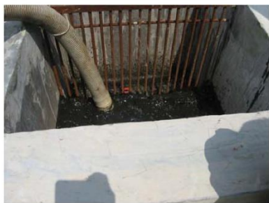
Sludge disposing from vagutug at Lakshmipur Pourashava
