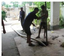
Sludge collection from septic tank with vagutug at Lakshmipur Pourashava
