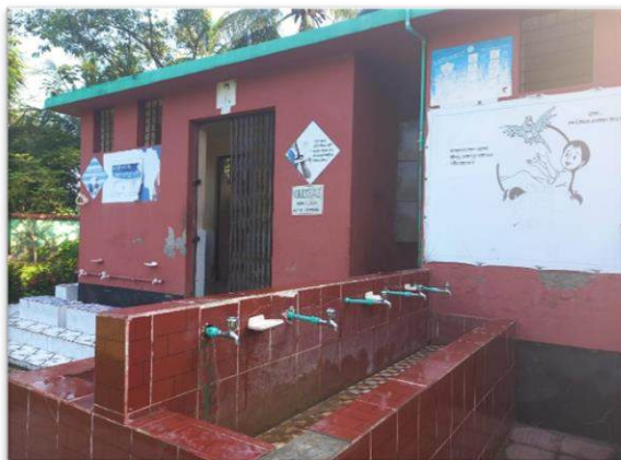
Figure 7: Photos of wash blocks that are not accessible for young children and children with disabilities
