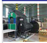
Horizontal External Furnace Waterstage Fired Steam Boiler
