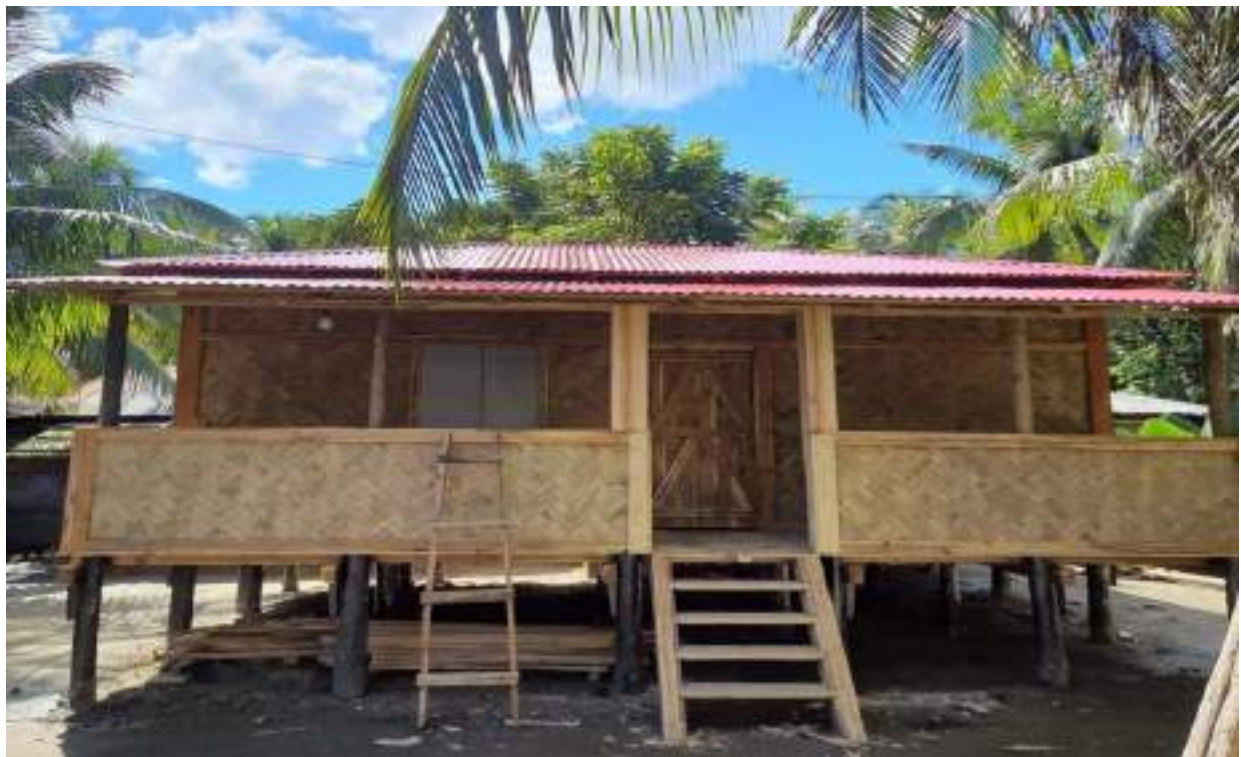
Specially Designed Machang House, Bandarban Hill District
