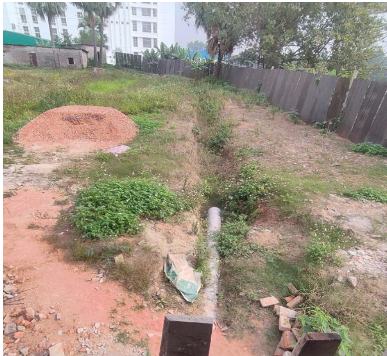
Figure 3-5 Drainage Line towards ETP
