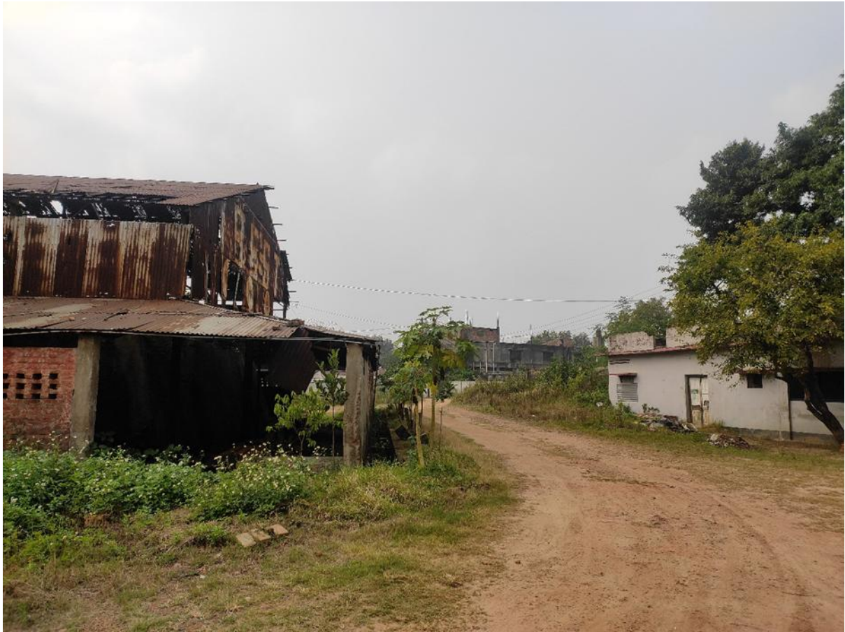
Figure 3-4 North side of the project
