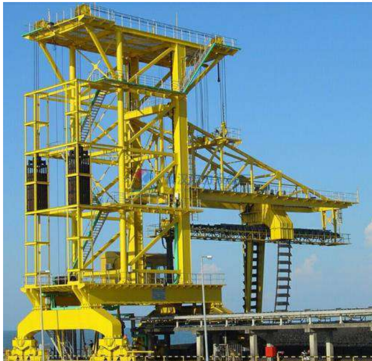
Figure 4-7: Catenary Chain Bucket Type Ship Unloader
