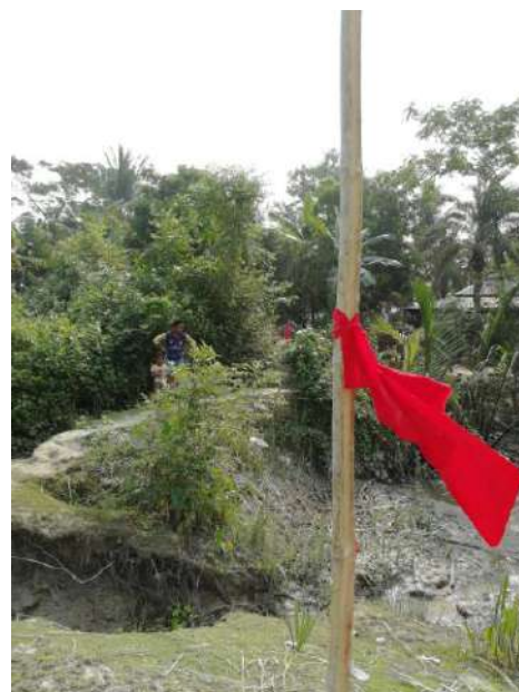
The west side of the project site
