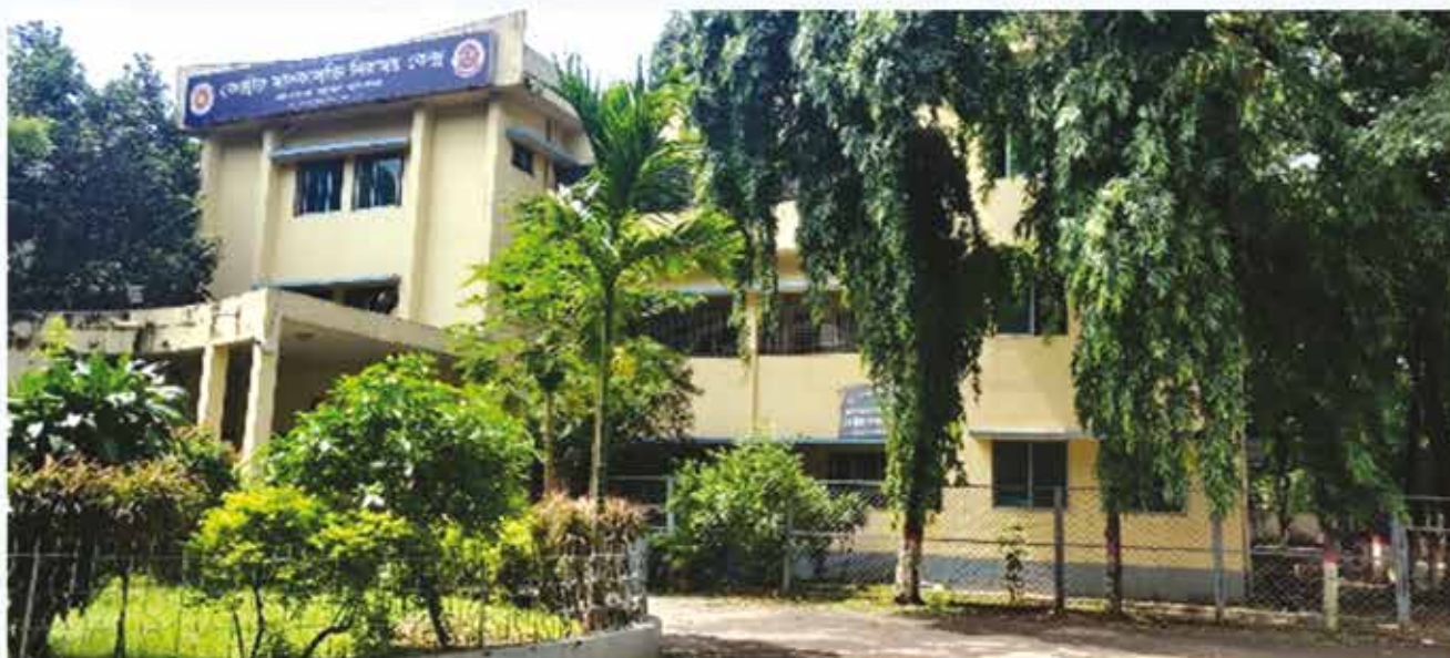
OST clinic at Central Drug Addiction Treatment Centre under the Department of Narcotics Control, Dhaka, Bangladesh
