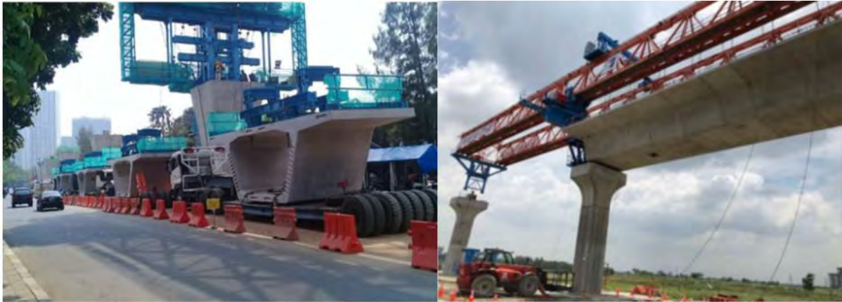
Figure 3-8: Span by Span Constructing Method
