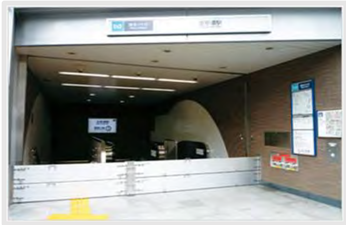
Figure 10-2: Flood Gate at the Entrance of Station
