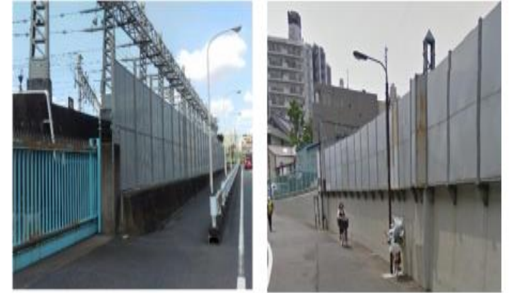
The height of walls have been raised.
