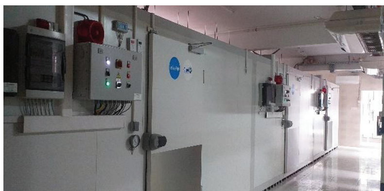
Newly installed WIC at Central EPI store
