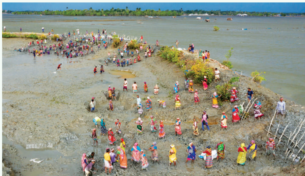
Man and woman work to repair damaged embankments after Cyclone Yaas struck Bangladesh in May 2021
