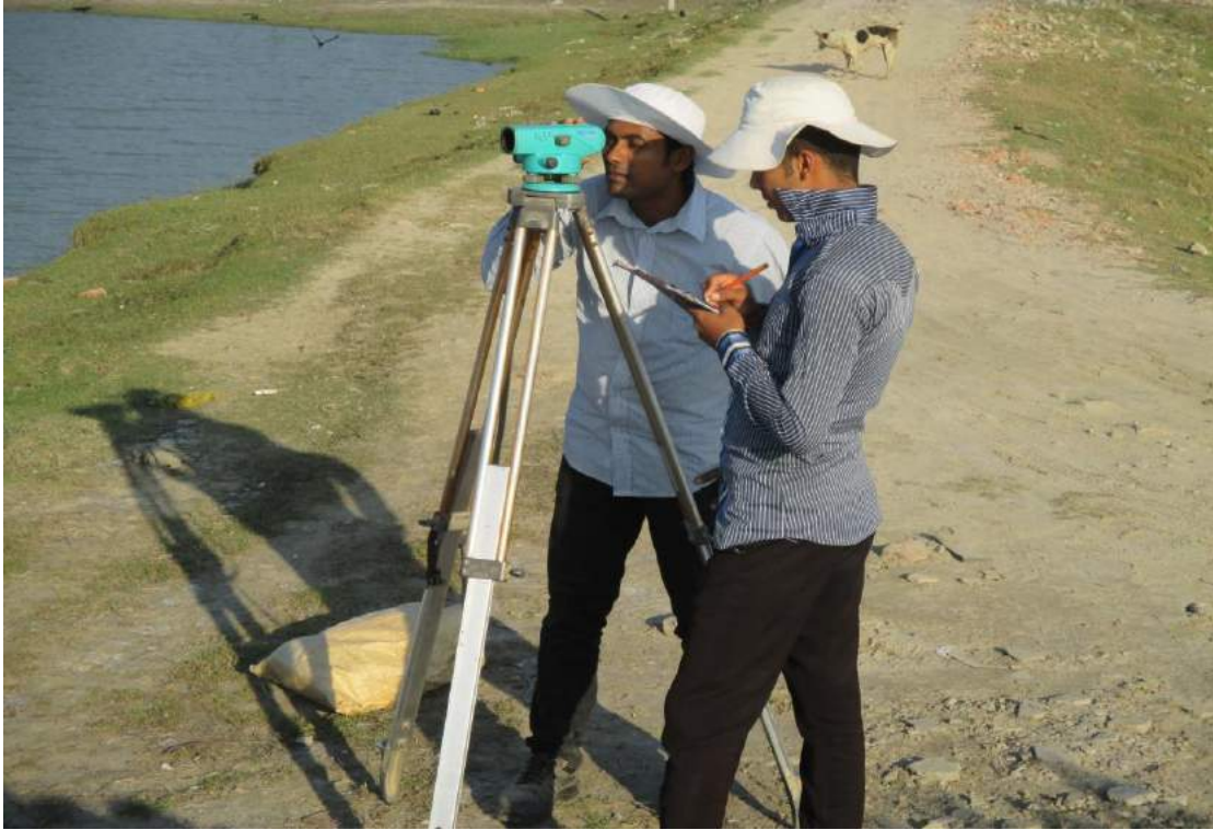
Figure 4: Checking the Heights With the Help of Digital Leveling Instrument
