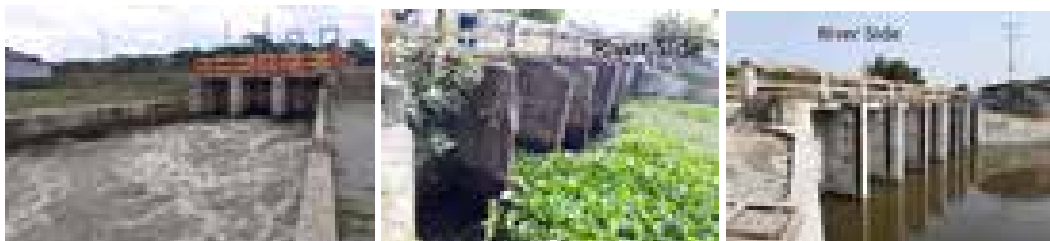
3-V Regulator constructed for better water management
