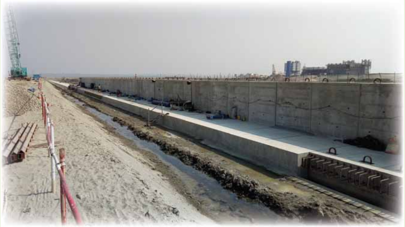
Matarbari 1200 MW USC CFPP L-Wall at Power Block Area
