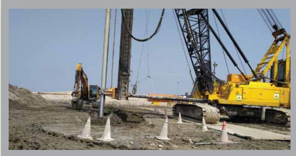
Deep Mixing Method (DMM) Works at Power Block Area
