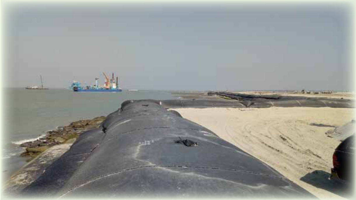
Geotex Bund (Sea Side) of Matarbari 1200MW USC Coal Fire Power Project
