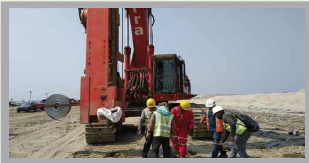
Pre-fabricated Vertical Drain Works at Power Block Area
