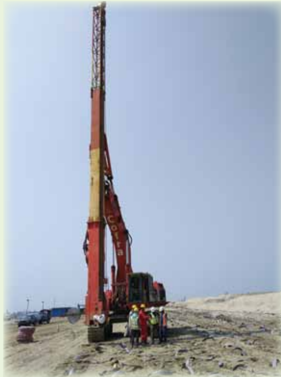
Matarbari 1200 MW USC CFPP PVD Works at Power Block Area
