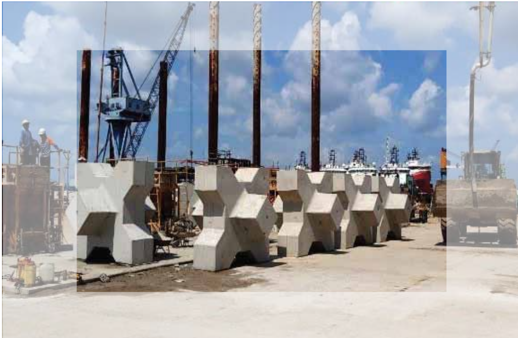
Fabrication of X-Block
