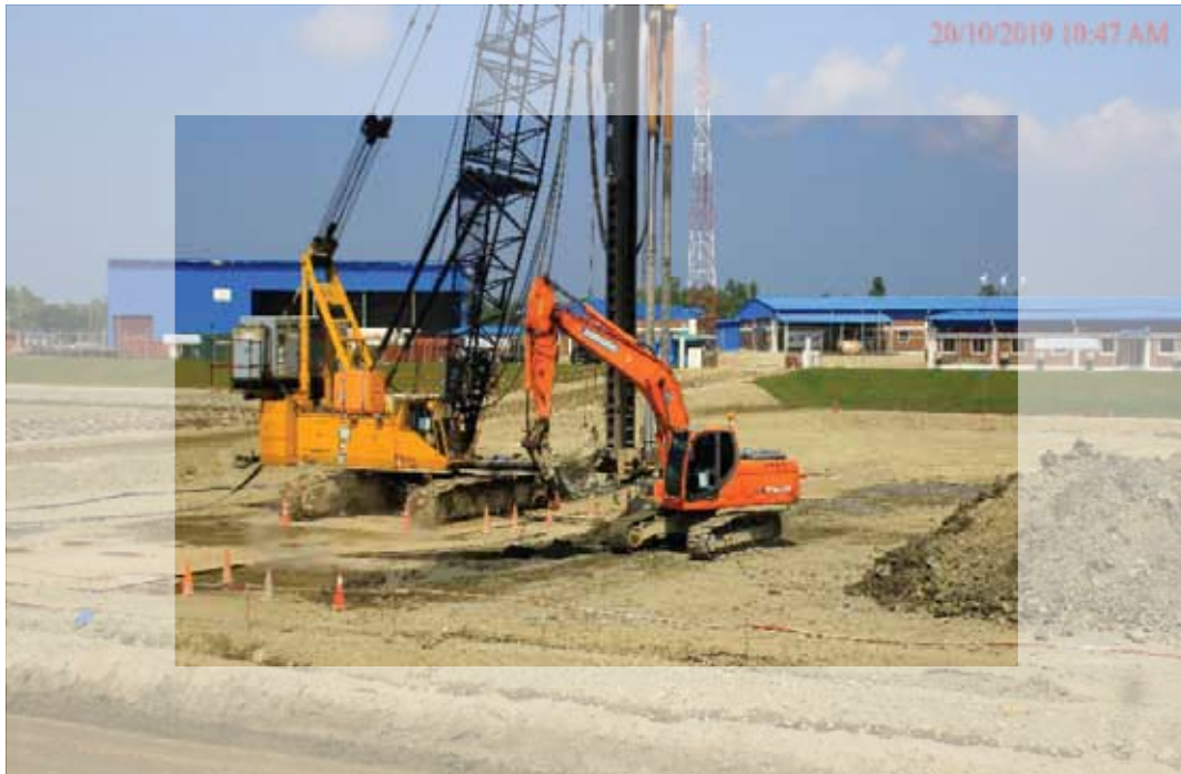
Soil Improvement - DMM Works
