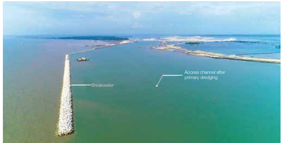
Breakwater is constructed to protect the access channel from wave and sedimentation
