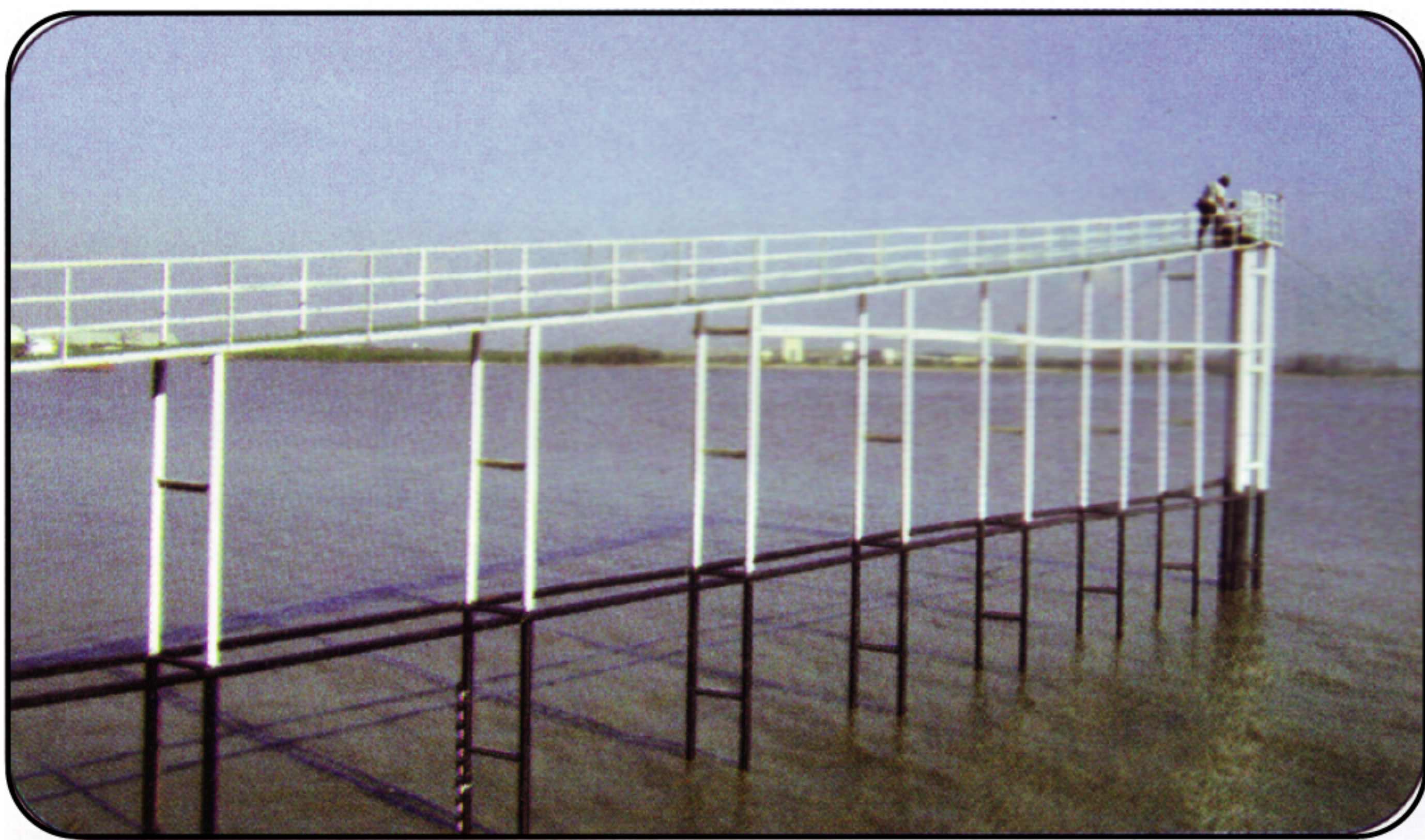
Auto Tide Gauge Station at Khal 18
