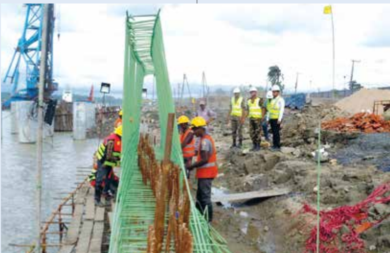
Breakwater is constructed to protect the access channel from wave and sedimentation
