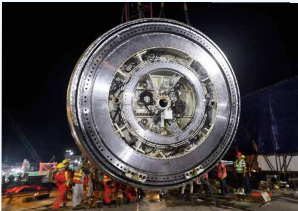
TBMs are used as an alternative to drilling and blasting (D&B) methods in rock and conventional 'hand mining' in soil
