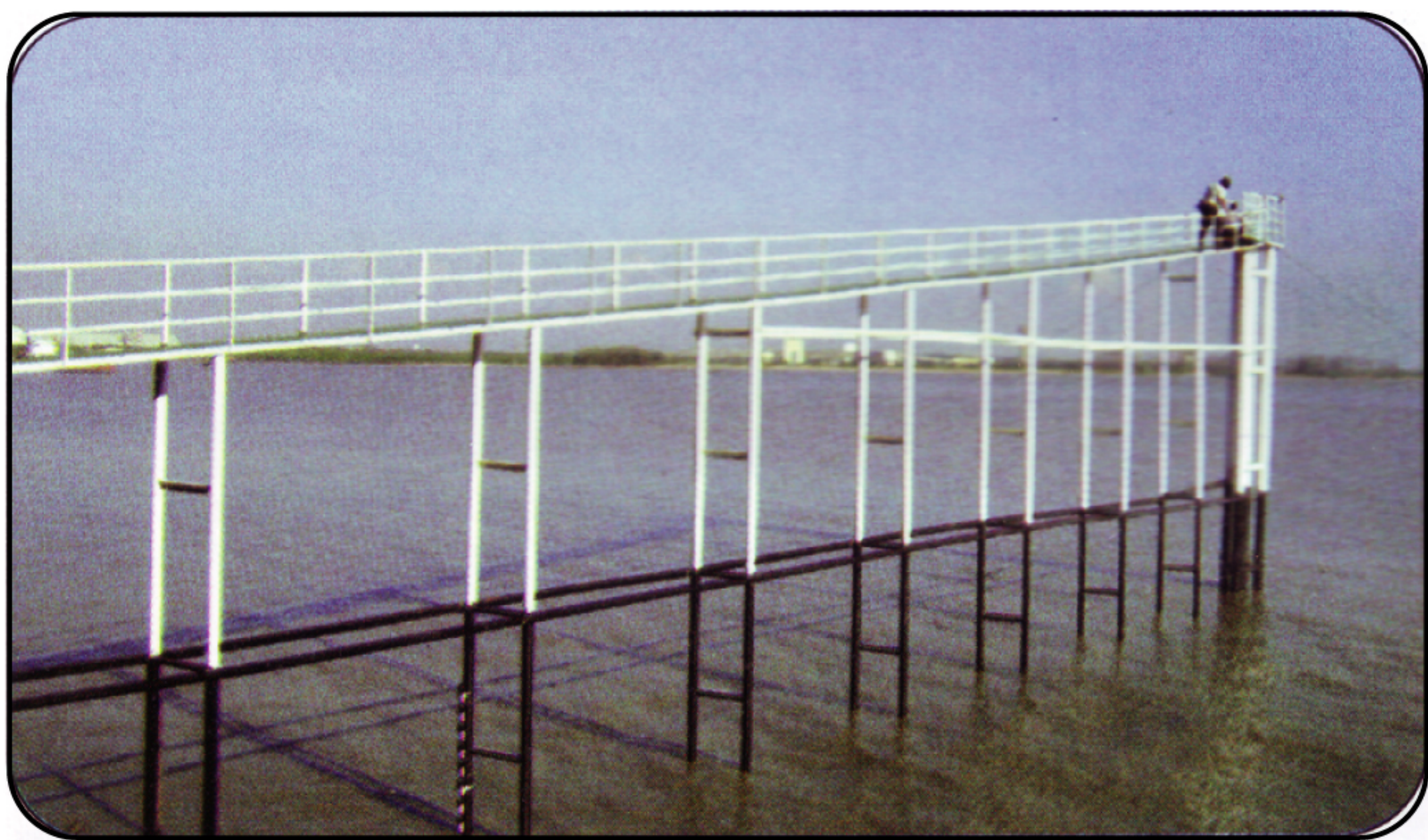
Auto Tide Gauge Station at Khal 18
