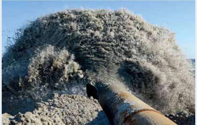
Silt is extracted down from the river bed and transferred to a different location through pipelines
