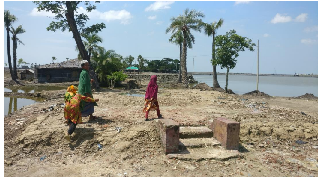
Sign of the effects of storm surge at ward no -3 (Date: 23.09.19)
