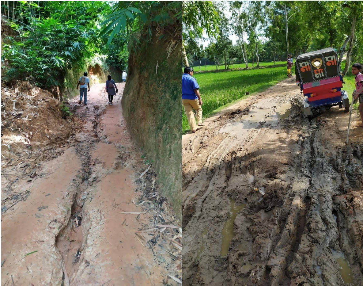
Figure 3: road to Jumpara from ward no 1 to 3 (left); road from ward 3 to 4 (right); both are prone to flood, flash flood.
