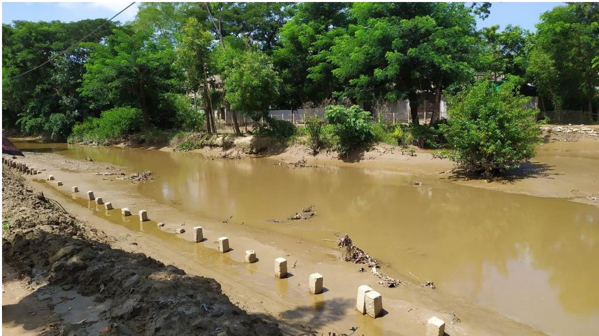
Figure 6: highly sedimented canal, this part flows through ward no 2 but the whole union is facing the same problem of siltation.
