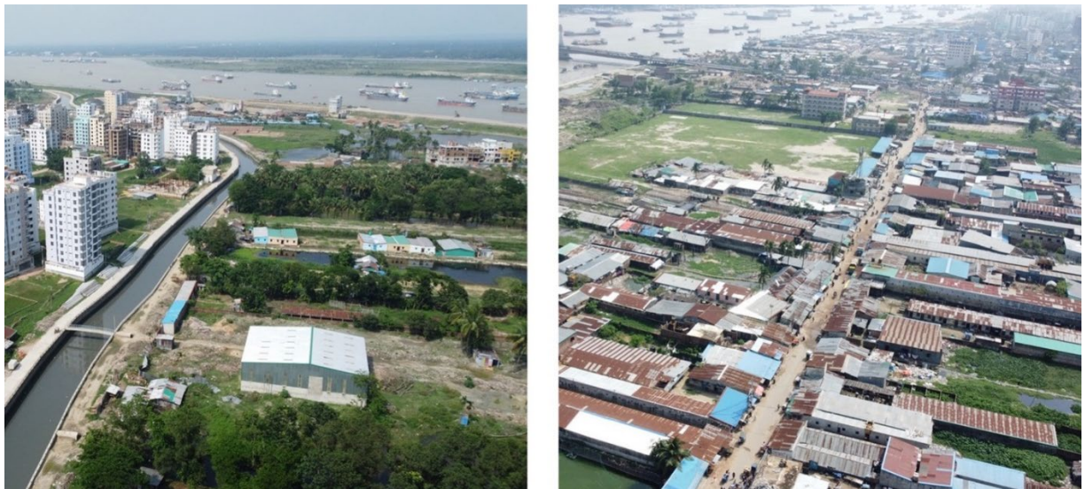
Figure 4: Existing Single Storied Structures in Bakalia
