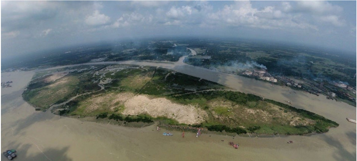
Figure 5: Existing Condition of Char Bakalia
