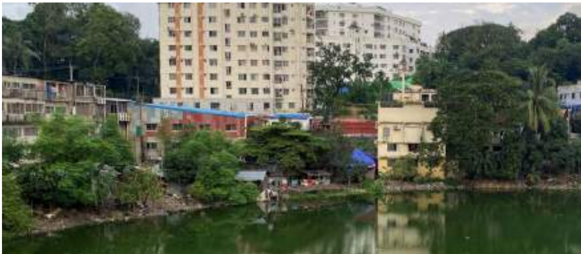
Figure 11-3: Unregulated Construction and Encroachment of Askar Dighi.
