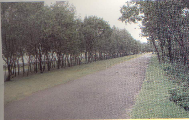
Pic. 4-6 Expansion of existing tree plantation zone can reduce vulnerability due to surges.
