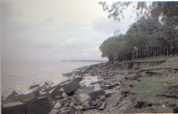
Pic. 4-7 Mangrove green belt may protect embankment from erosion.
