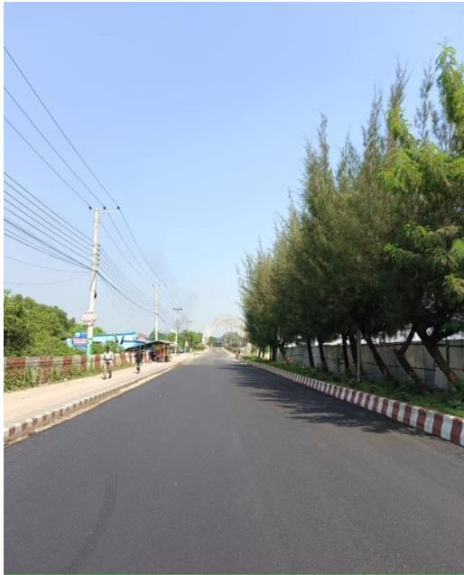
Airport VIP Road , Finishing Work
