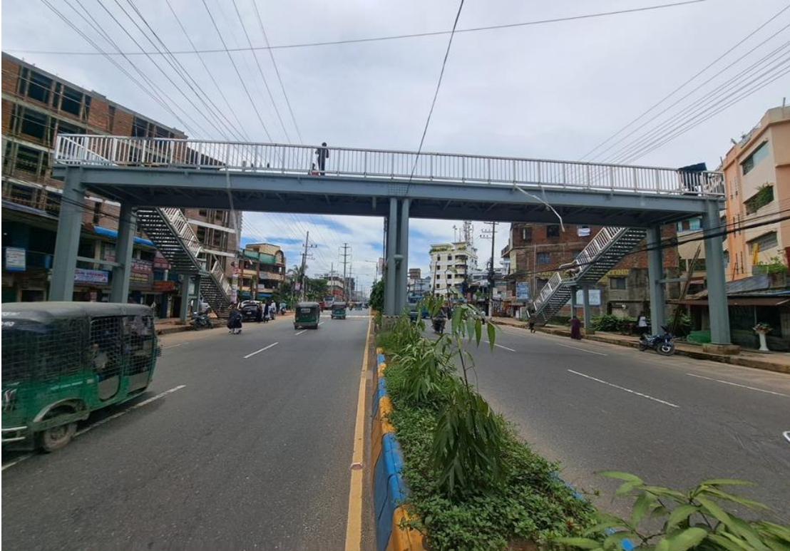
Foot Over Bridge , Running Work
