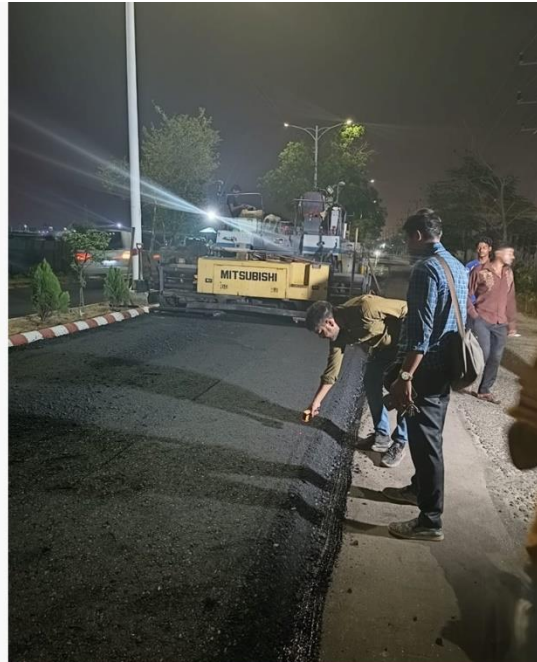
Airport VIP Road, Running Work
