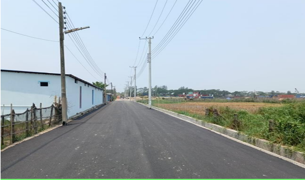
Golichipa Road Finishing Work
