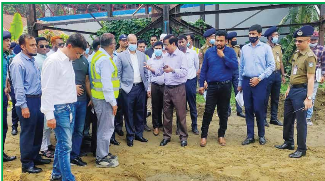
In time of inspection of the Multi-Modal Containet Terminal under construction at Haliashahar, Chottogram.
