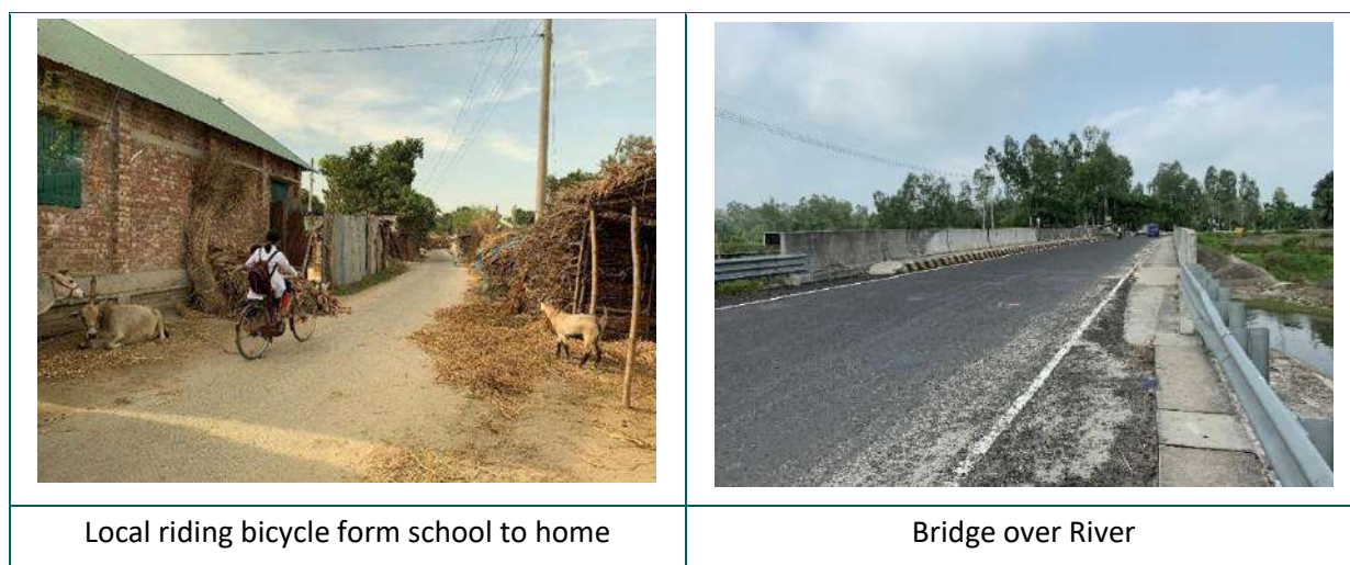
Figure 5-14: Pictures of Communication Facilities
