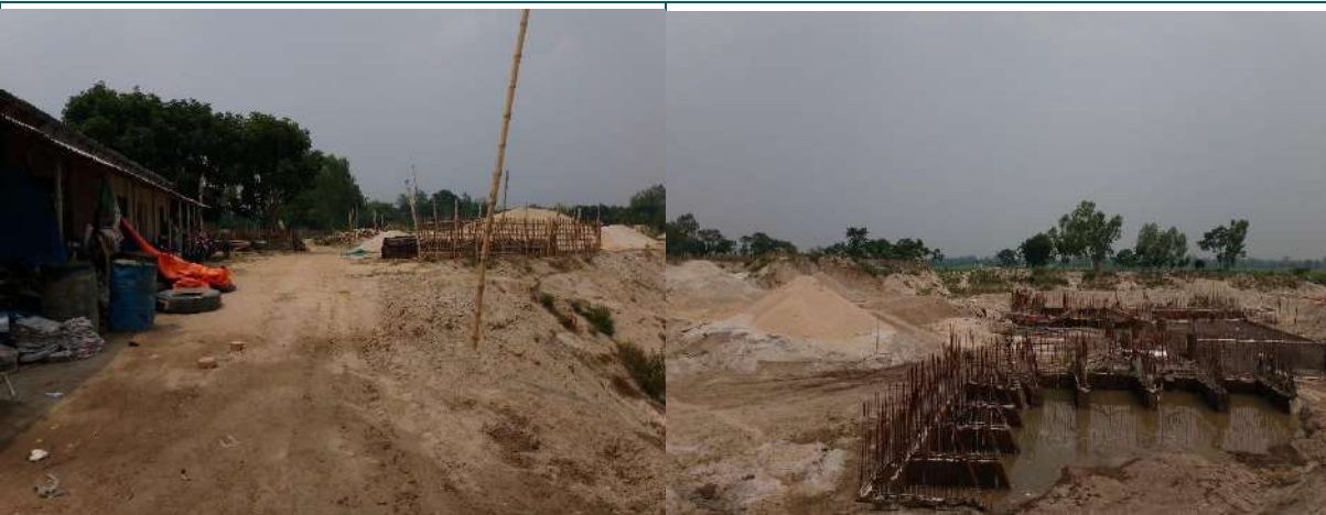
Combined Water Control Structure at Beltola over Shuk River
