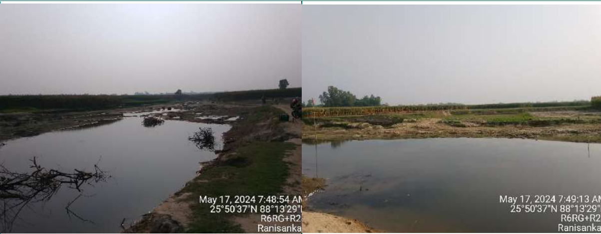
Combined Water Control Structure at Rautnagar over Kulic River
