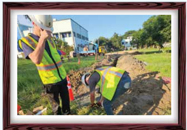
SMW-6 land cable installation at Cox's bazar landing station.
