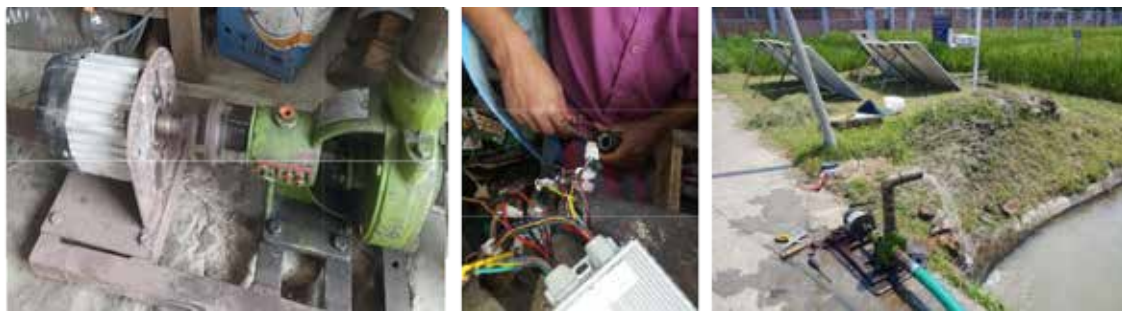
Fig.6: Installation of DC solar irrigation pump.
