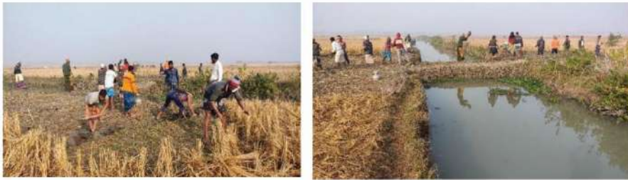
Fig. 11. Trapped fresh water by earthen embankment, Dacope, Khulna, Rab, 2021-22.
