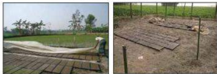
Photo 10 Tray covered by polyethylene and fencing
