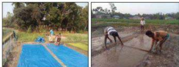
Photo 24 Placement of mud and leveling
