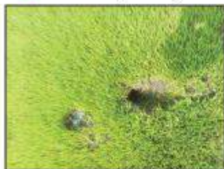
Photo 28 Mat damage by rodents and excessive soil height
