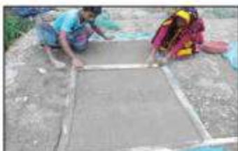
Photo 20 Leveling the soil
