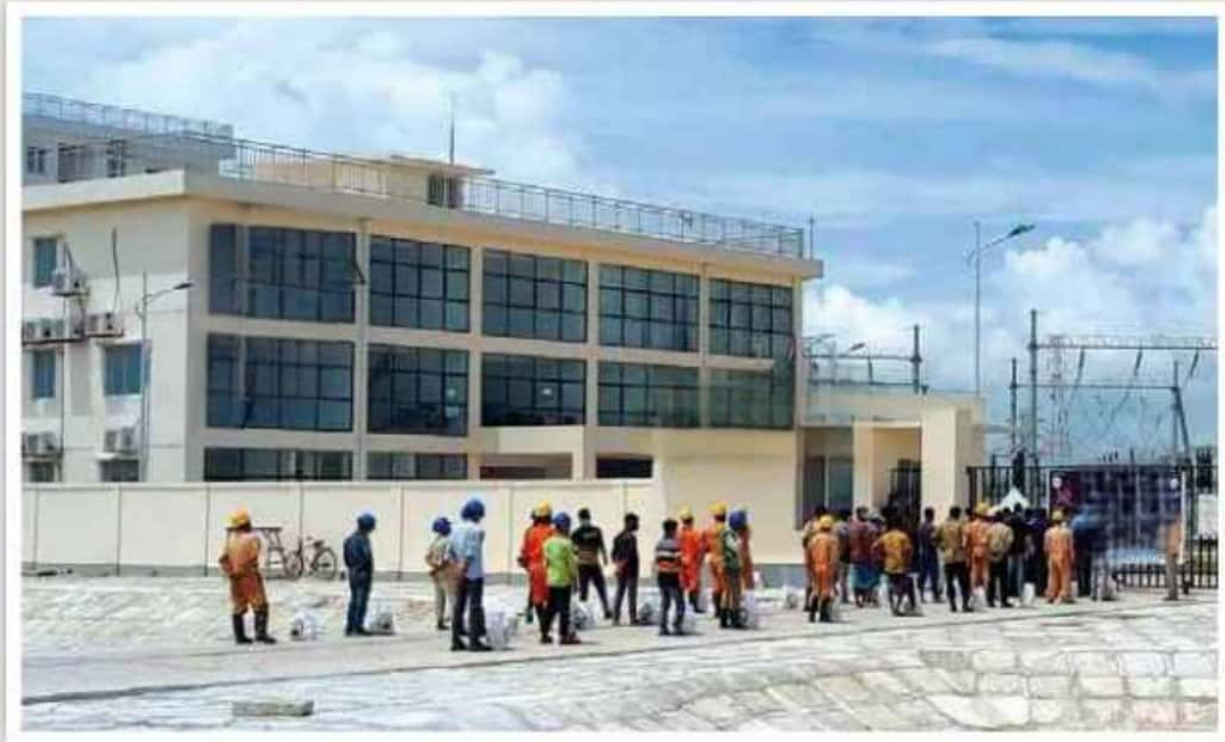
Food Aid Program at Mirsarai 150 MW Dual Fuel Power Plant Project
