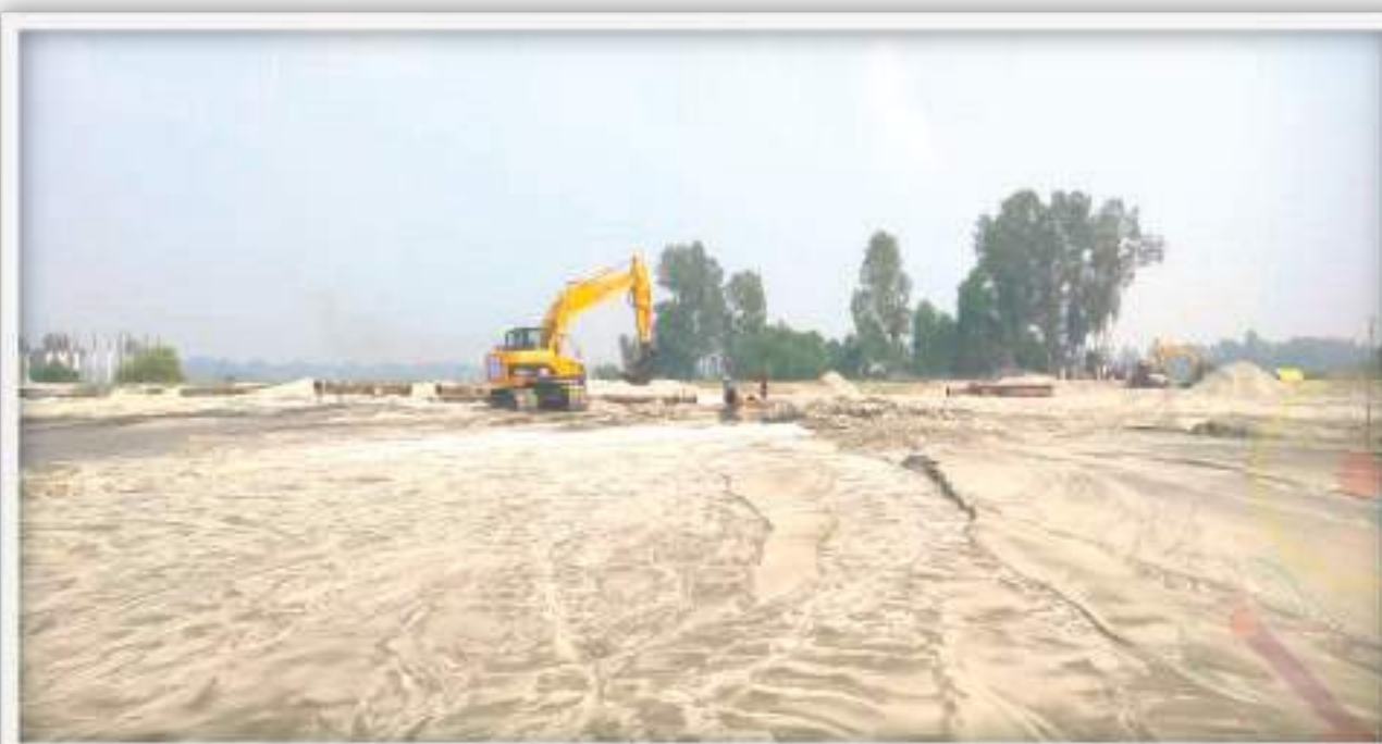
Sand filling at Madarganj 100 MW Solar PV Power Plant Project
