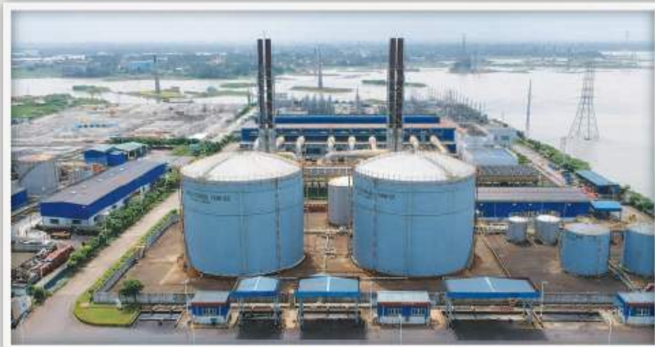
Kodda 150 MW Power Plant
