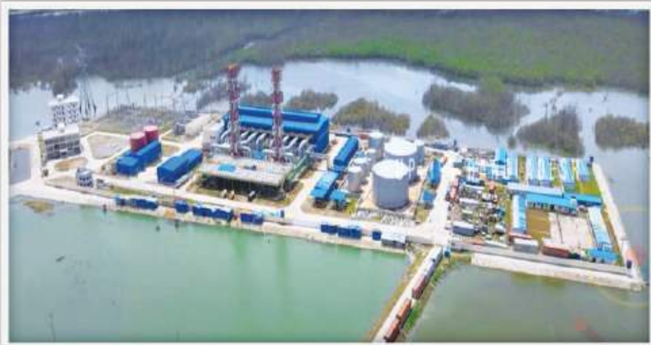
Mirsarai 163 MW Dual Fuel (HFO/Gas) Power Plant
