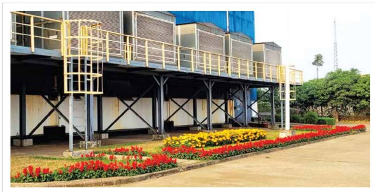
Beautification of Kodda 150 MW Power Plant
