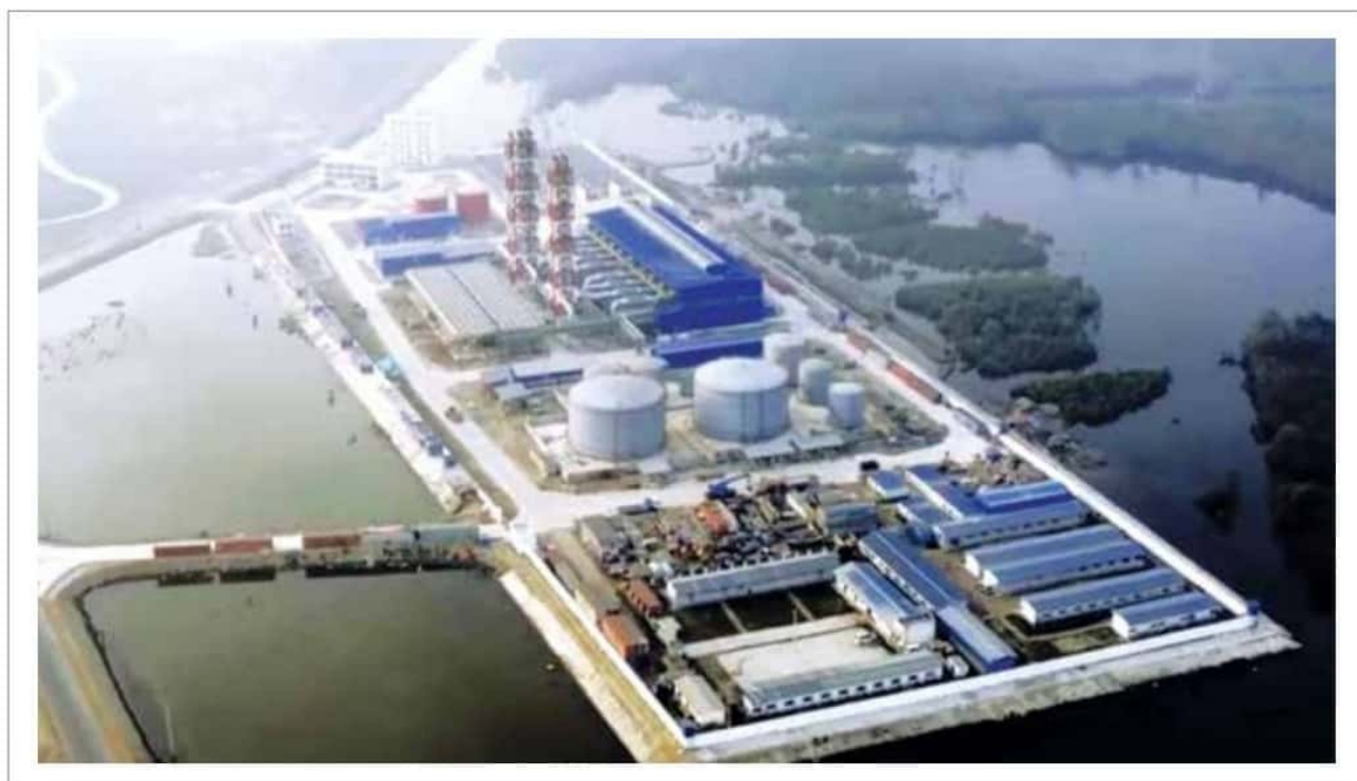
Mirsarai 150 ( \pm 10\% ) MW Dual Fuel (Gas/HFO) Power Plant Project Overview.
