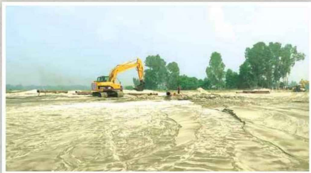
Land Development of Madarganj 100 MW Solar Power Plant Project
