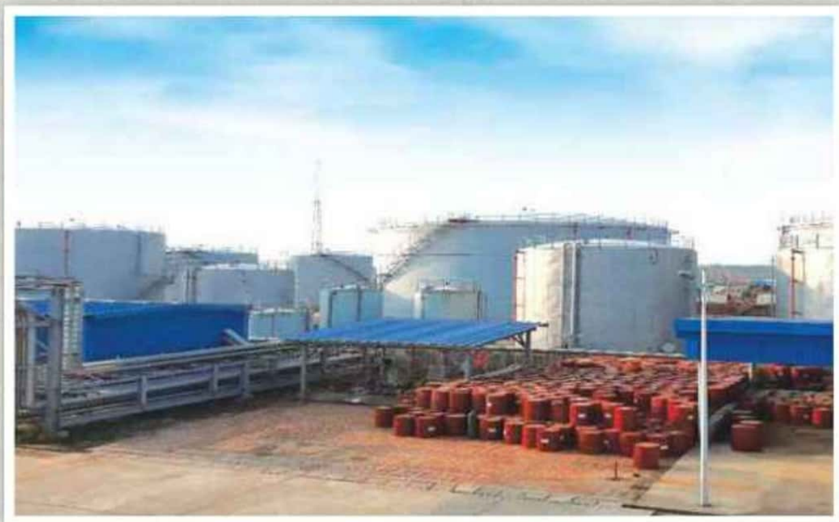
Mirsarai 163 MW Dual Fuel (HFO/Gas) Power Plant
