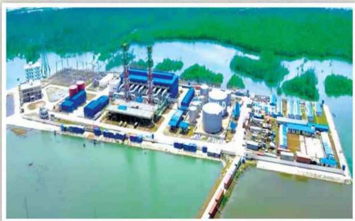
Mirsarai 163 MW Dual Fuel (HFO/Gas) Power Plant
