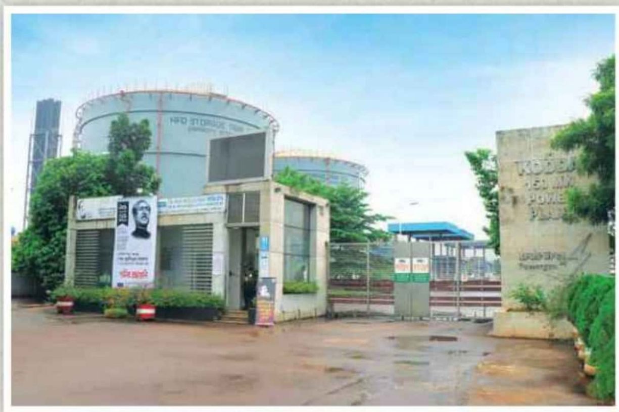
Kodda 150 MW Power Plant
