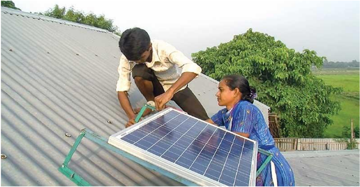
Fig 1. Installing PV cell at a house in a rural area.
