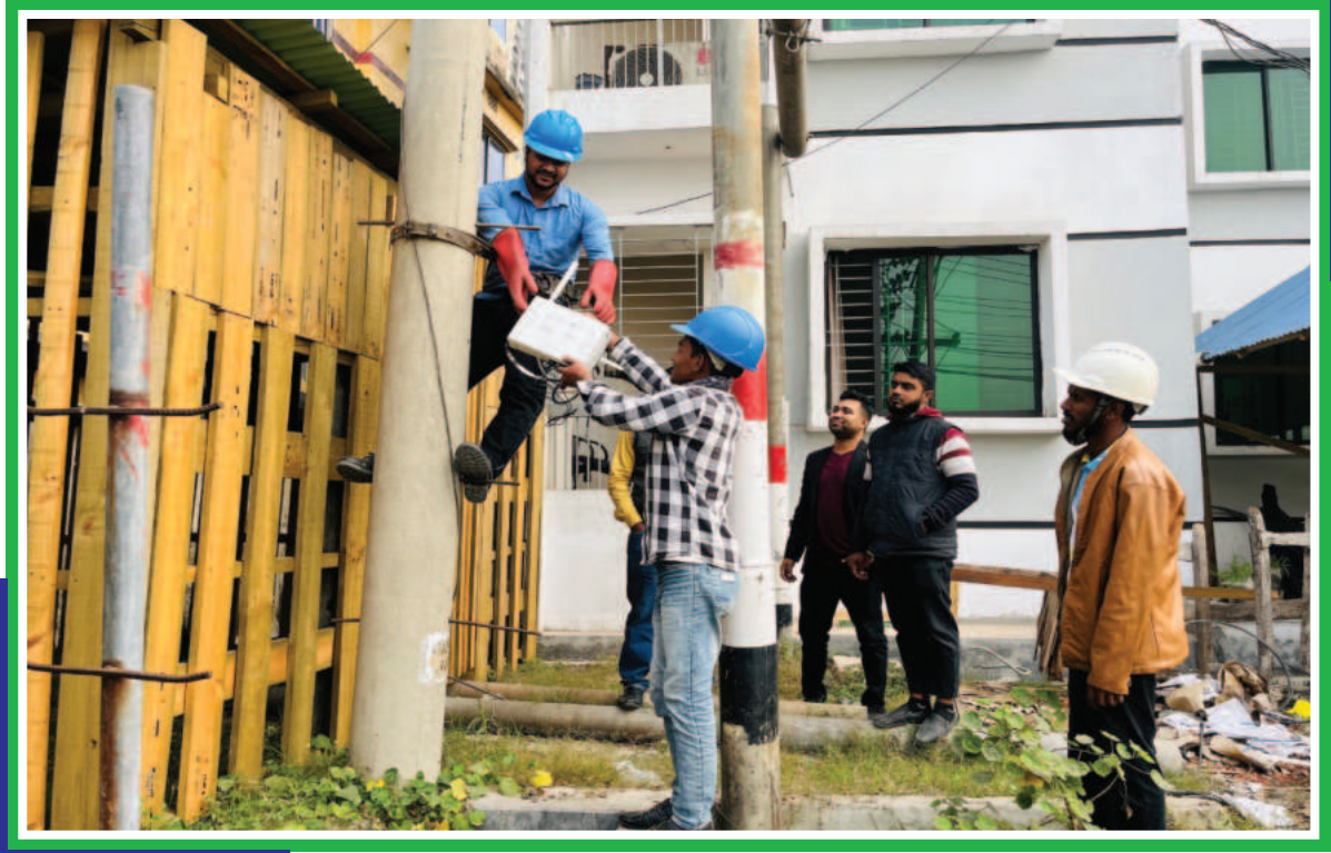
DCU Installation Work at Dhaka PBS-4
