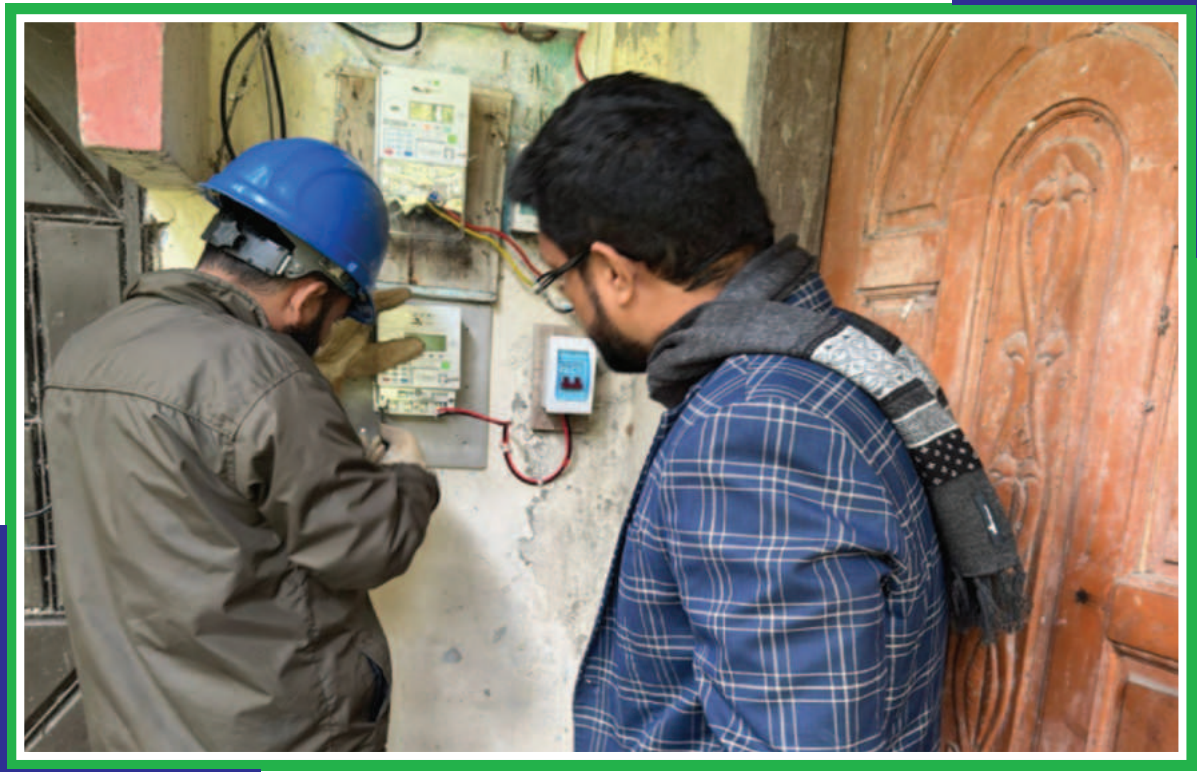
SPPM Installation Work at Dhaka PBS-4
