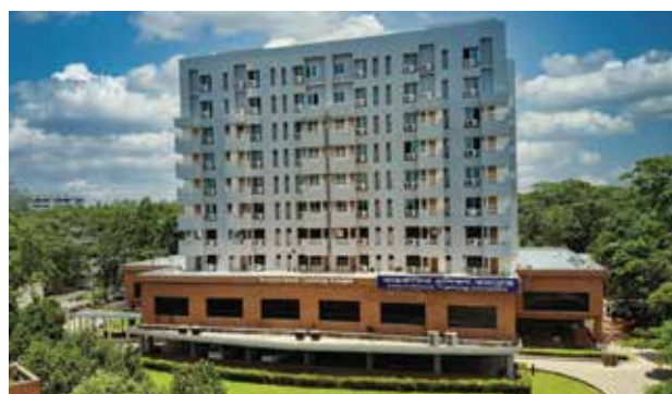
ITC building; after the completion of vertical extension
