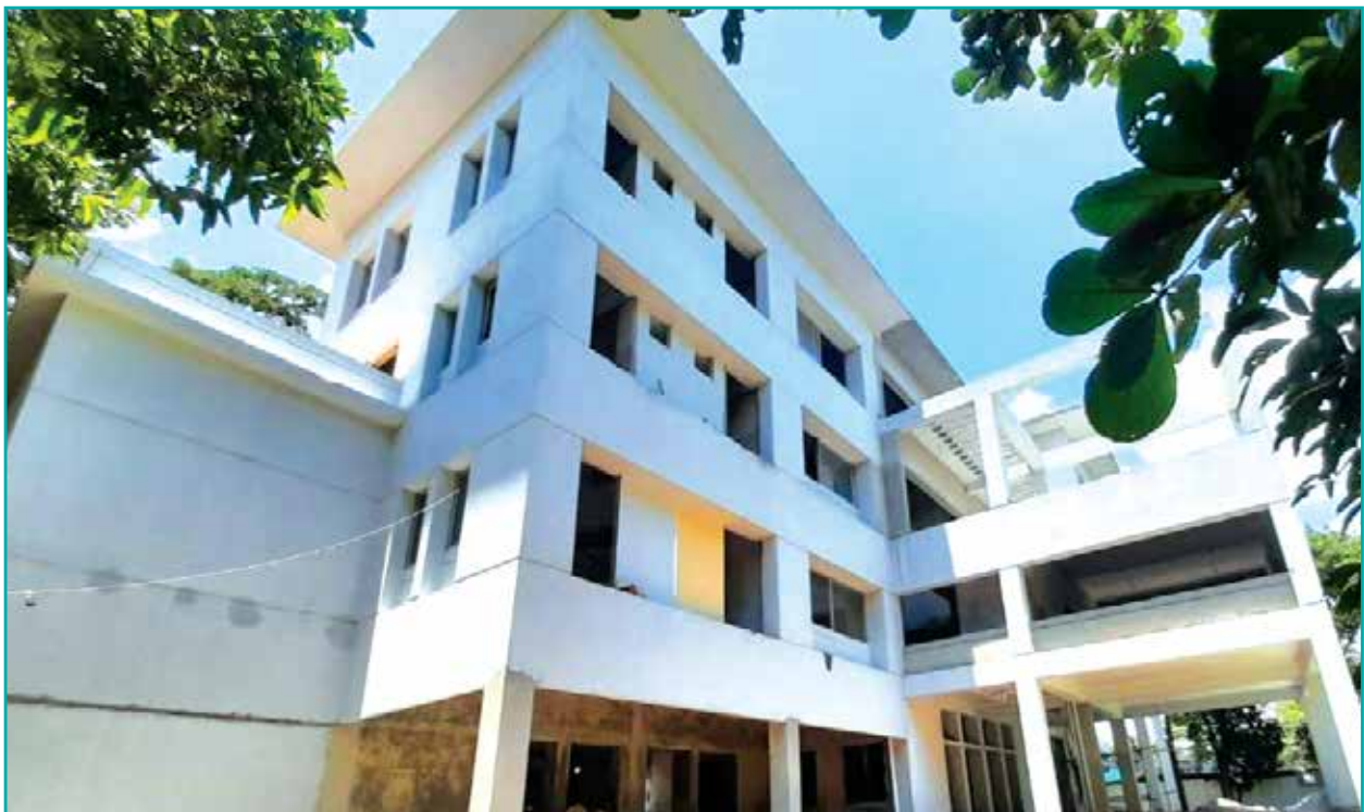
4 -Storey BPATC Clinic
