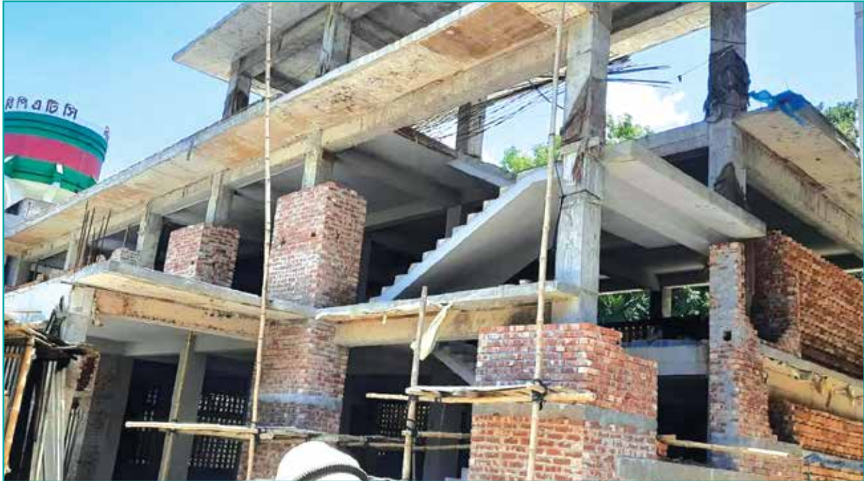
Work in progress of a two-storied substation building
