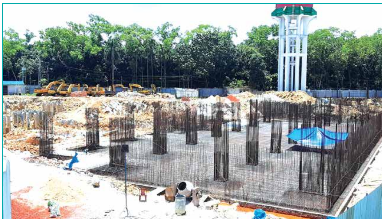
Pile Cap Casting of 20 storeyed Bangabandhu Sheikh Mujib Academic-cum-Administrative Building
