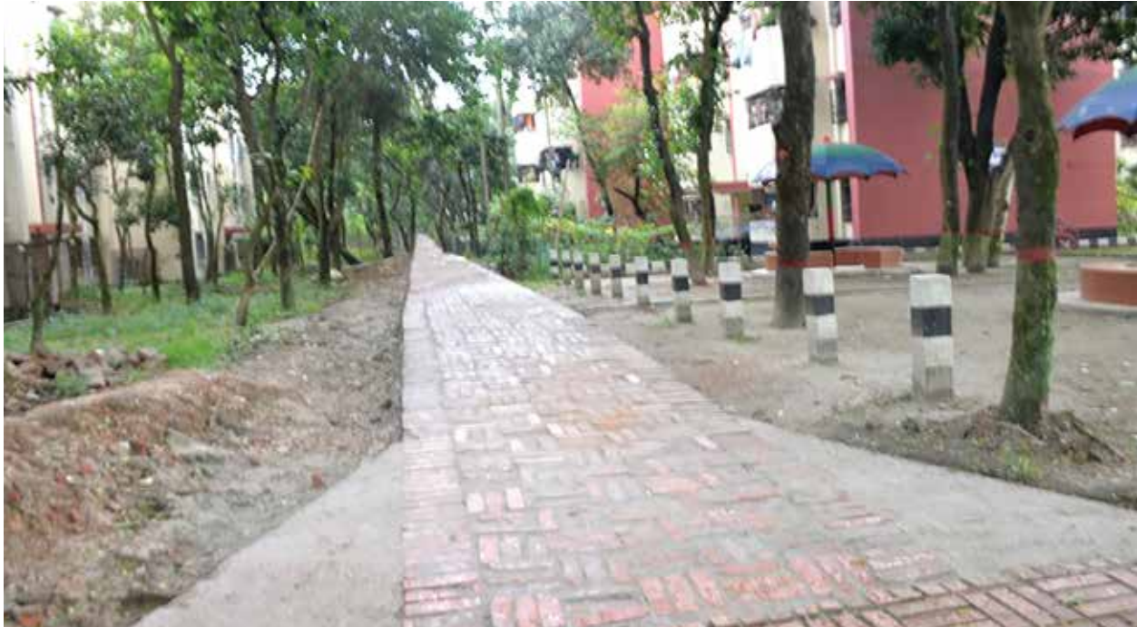
Renovation of internal roads and footpaths between the residential buildings
