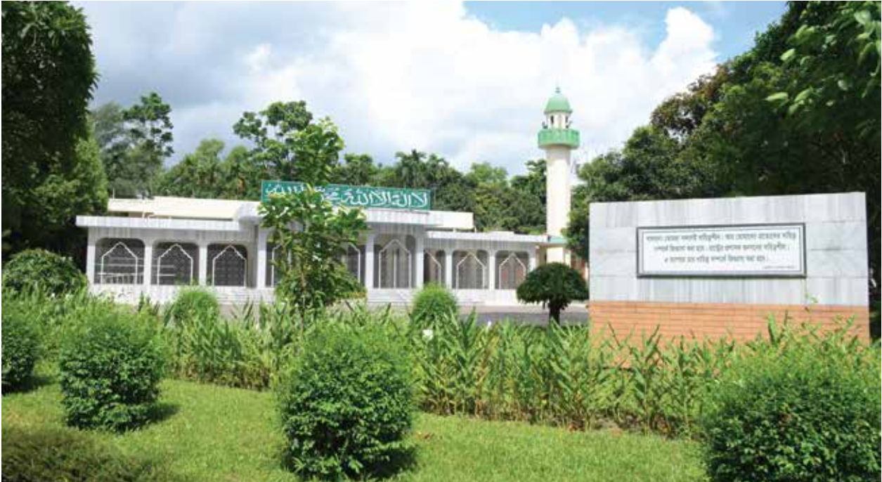
A view of renovated Mosque of BPATC
