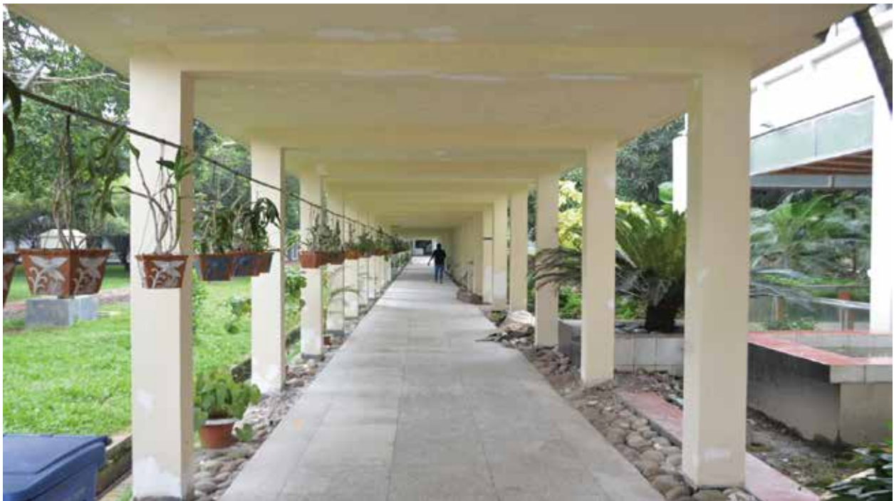
Renovated Corridor of the centre
