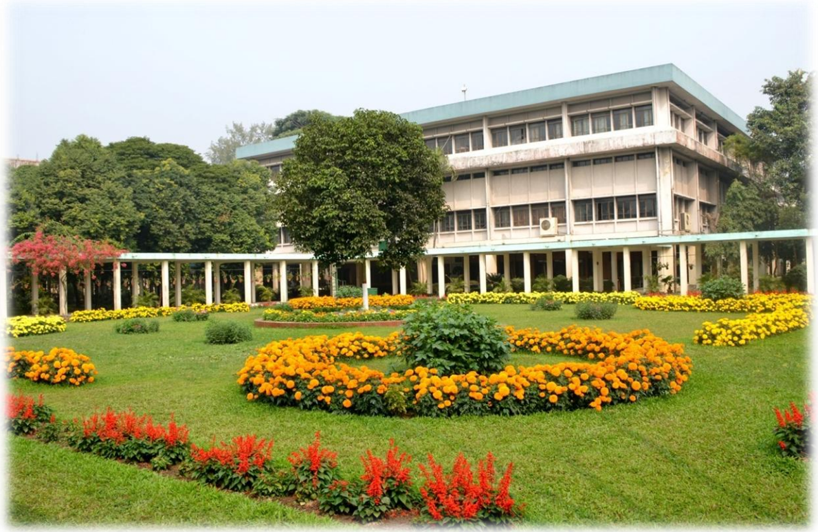
Library Building of BPATC
