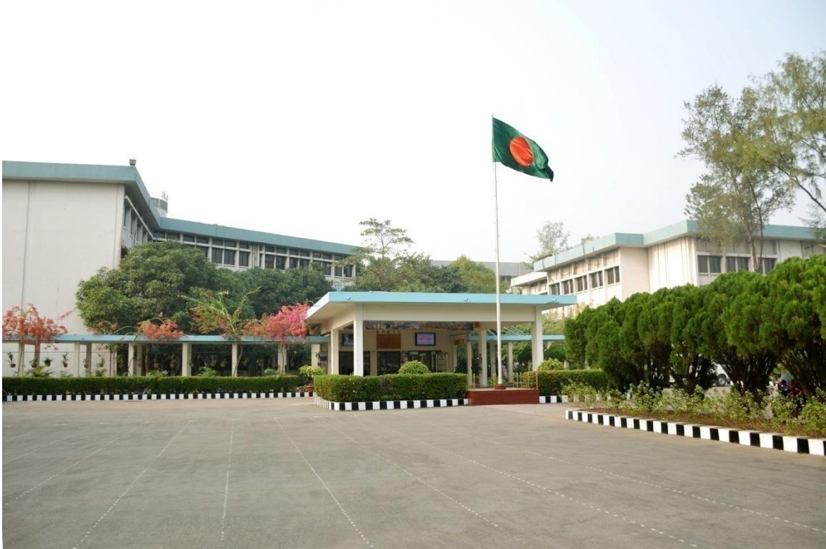
BPATC Main Reception, Administrative and Syndicate Building
