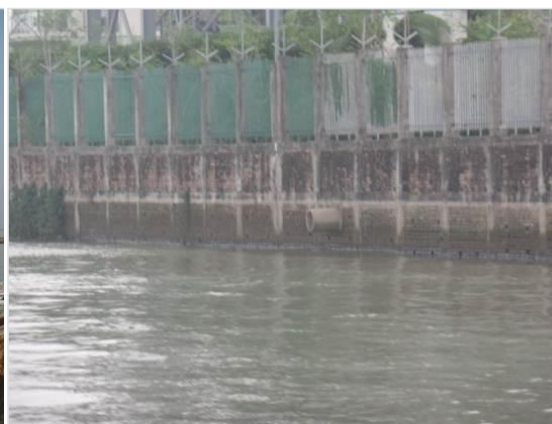
Figure 5-34: Surface water pollution source in the project influence area
