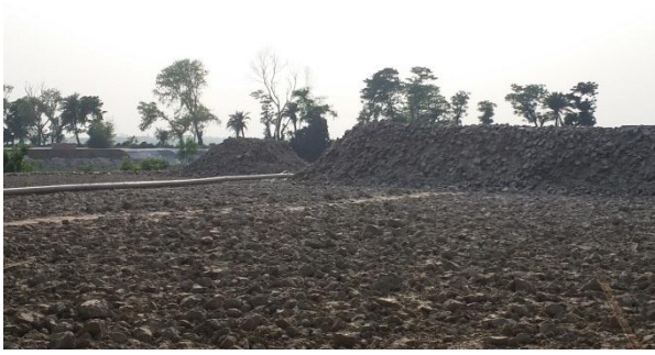
Figure 12-19: Filling up of low laying areas with dredge materials by private operators at Location 2 (Selimabad)
