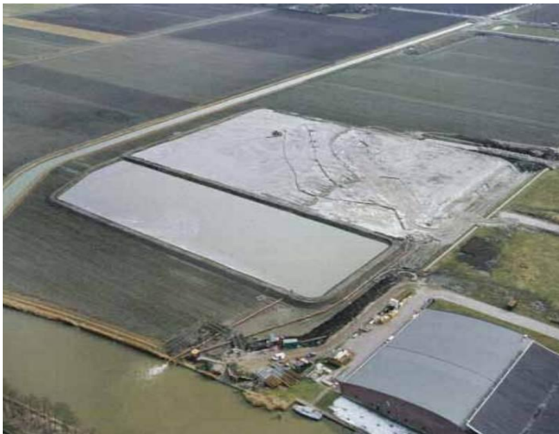
Figure 10-5: Disposal Area with Silt Pond
